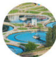
Sewage / Effluent Treatment Plant
