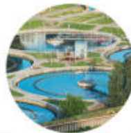
Sewage / Effluent Treatment Plant
