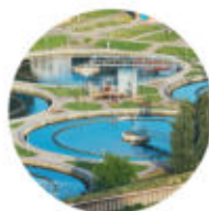
Sewage / Effluent Treatment Plant
