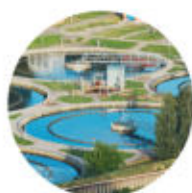
Sewage / Effluent Treatment Plant
